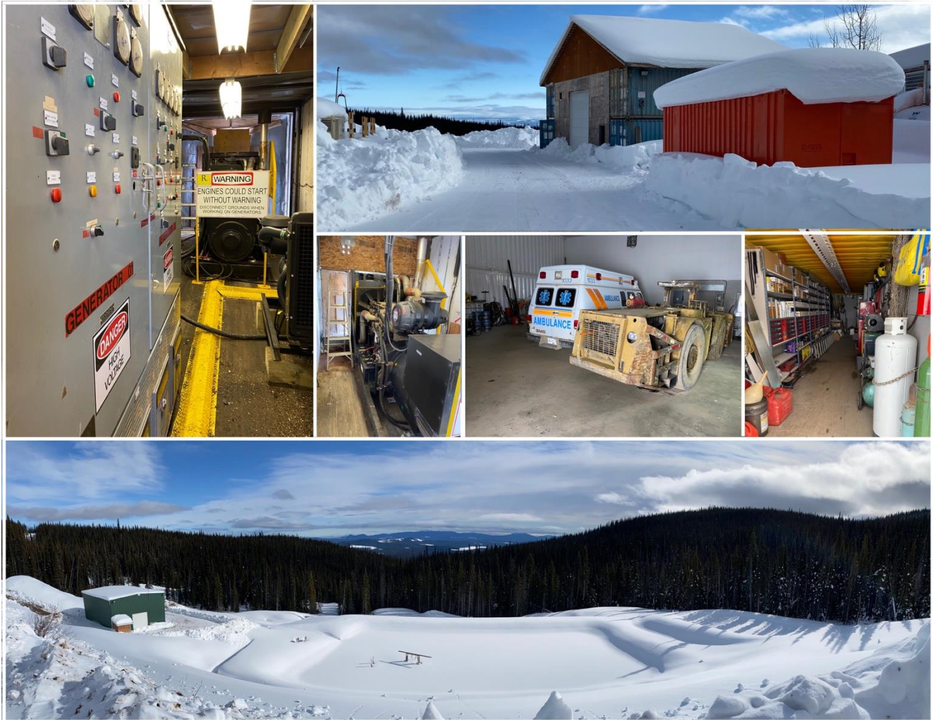
Dome Mountain Mine is efficiently designed and well maintained.
