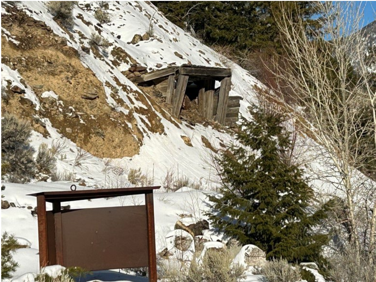
Figure 4.3. View of 360 Level Portal Source: Photo by AMPL, 2025
