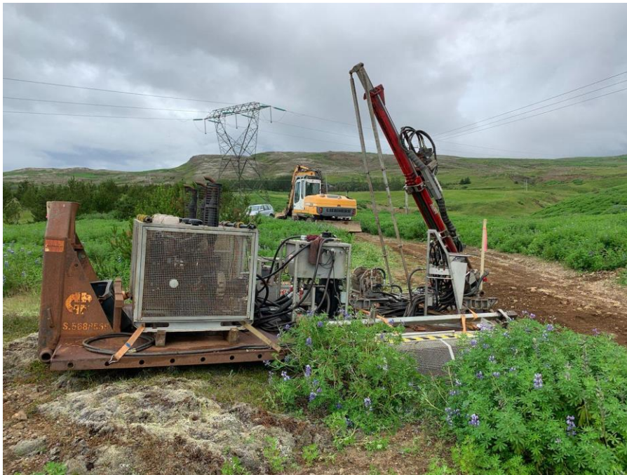
Picture 1. Drill Rig on Thor Gold Project
