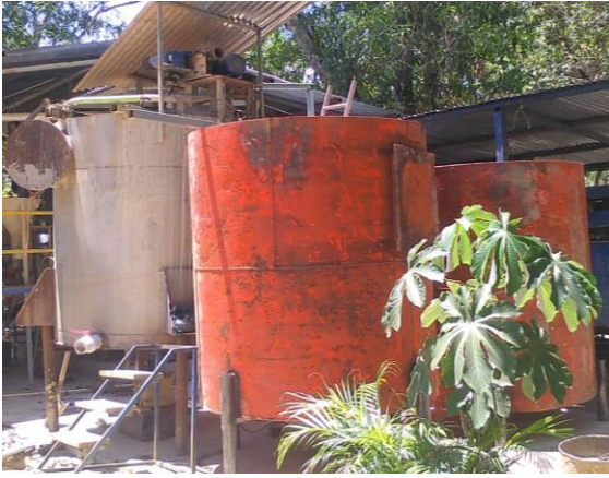
Figure 2. Fabrication of New Tanks
