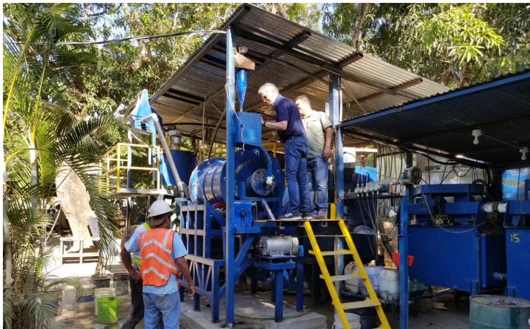
Figure 1. Management Inspecting Plant Upgrades
