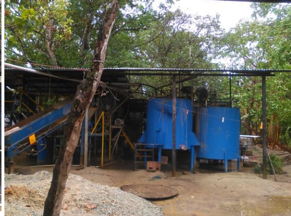
Figure 3. New Tanks Completed
