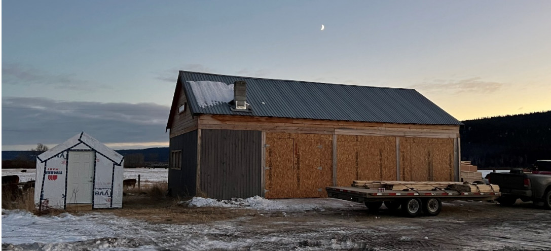
Carlyle Commodities Core Logging and Processing Facility
